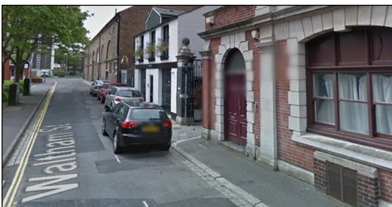
Waltham Street entrance to rear communal area of Charter House and Beddow Hall (location of waste bins and fire escape)
