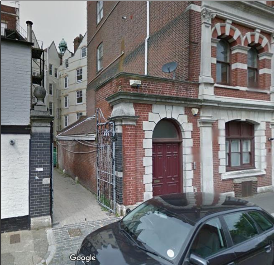
Access to rear communal area of Charter House and Beddow Hall, via Waltham Street entrance
